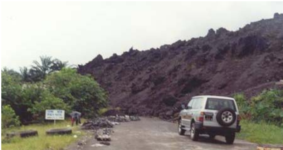
Picture 4: Blockage made to roads infrastructure at Bakingili on the way to Idenau during Lava flow of 1999
