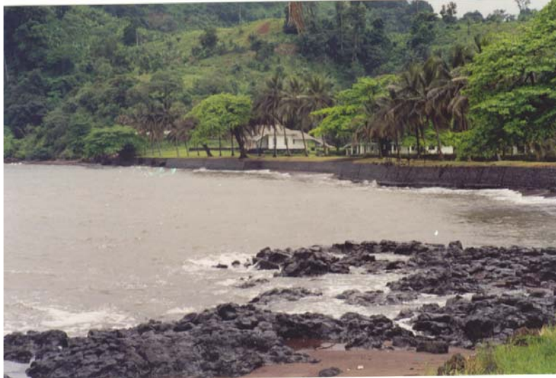
Picture 14: Bota – Limbe beach with volcanic rocks in front of catholic eathedral with beach protection built opposite.
