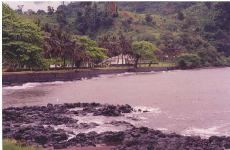
Picture 15: Bota – Limbe volcanic rocky beach opposite protective wall against erosion
